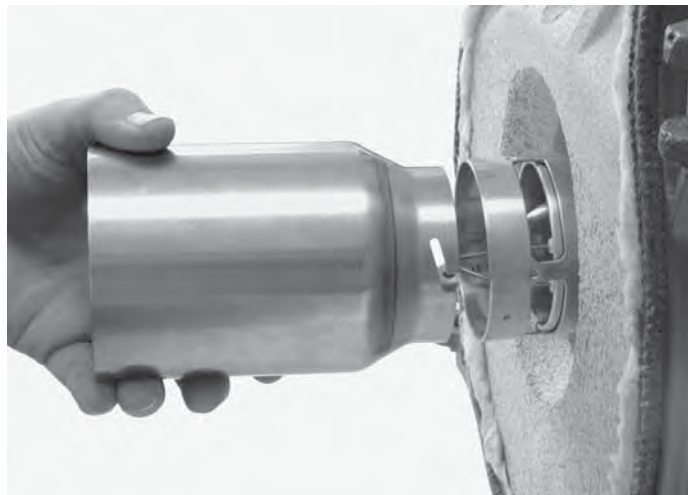
The re-circulation openings should not be covered by the insulation of the combustion chamber.
